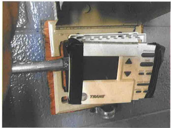
FIGURE 3 - EXISTING THERMOSTAT TO BE REPLACED
