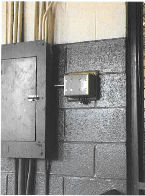
FIGURE 3 - EXISTING THERMOSTAT TO BE REPLACED
